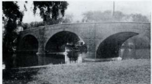
Bridge Erected in 1799 and Spanning Periomon Creek, Near Collegeville, Pennsylvania. The Stone is Pennsylvania Sandstone. The Upper Portions Have Been Rebuilt of the Same Stone.
