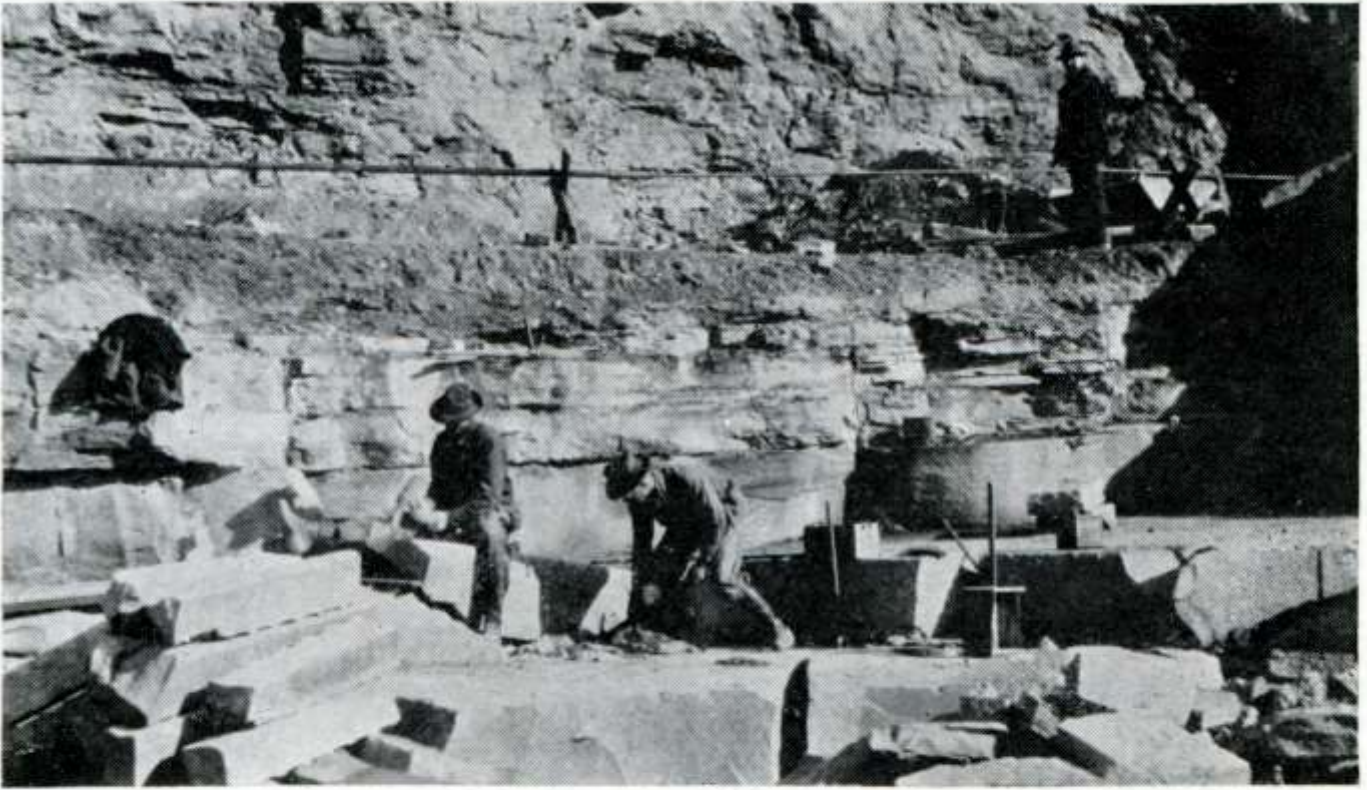
Sandstone Quarry near Waynesburg, Greene County, Pennsylvania, Showing Brick Shale in Upper Strata Being Worked in Advance of Dimension Stone Operation Below.
