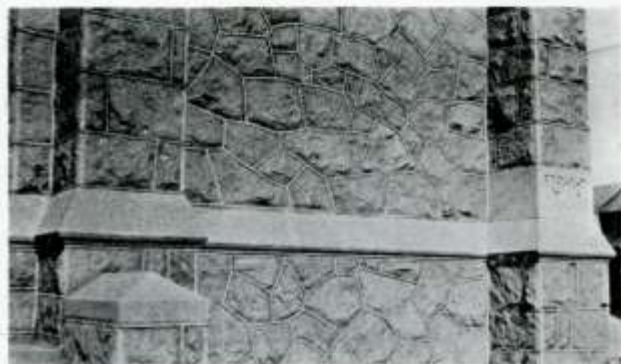
Seisholtzville Granite in St. John's Lutheran Church, Emaus, Lehigh County, Pa., Erected in 1923. This detail shows a masonry wall of unusual rustic beauty.
