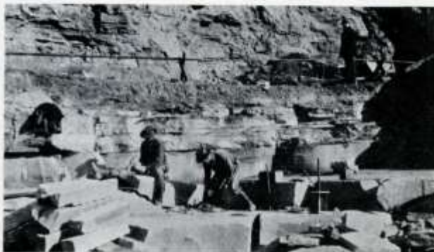
Sandstone Quarry near Waynesburg, Greene County, Pennsylvania, Showing Brick Shale in Upper Strata Being Worked in Advance of Dimension Stone Operation Below.
